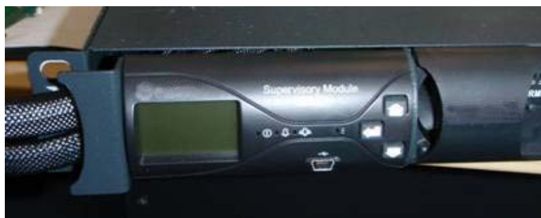
Fig 6. For removal, pull monitor forward to release the ball catch
